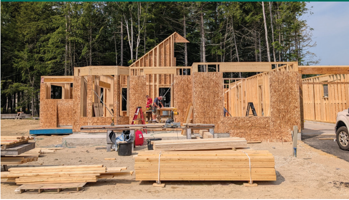
True North Builders work on a cottage on Monarch Drive in Phase 2 of Cumberland Crossing. (8/8/25)
