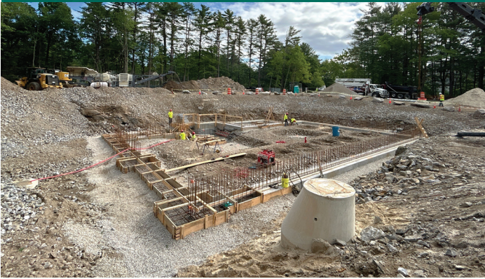
A view of Building C on 6/20/25. (Photo courtesy of Zachau Construction.)
