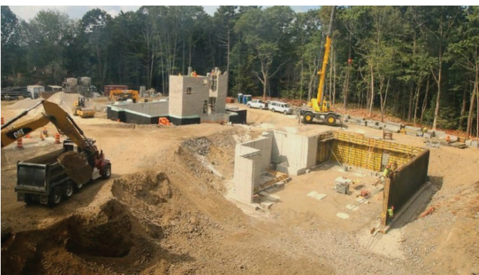
The view from our construction cam. Foreground: Building B. Background: Building C. (8/15/25)
