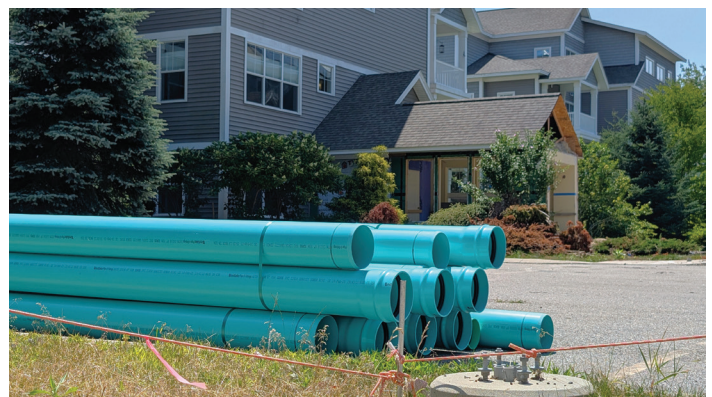
A view of construction at the Blueberry Commons Expansion. (7/24/25)
