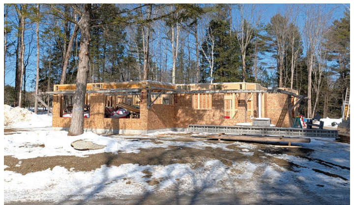
Construction in Phase 2C of Cumberland Crossing. (02/27/26)
