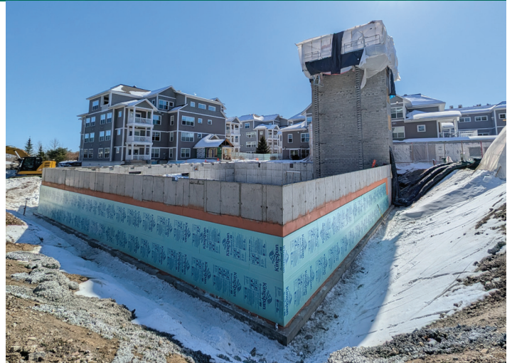
Blueberry Commons Expansion under construction. (02/27/26)
